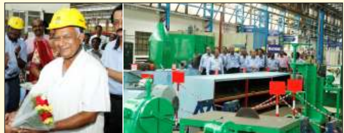
Renovated Electrical Shop was inaugurated by Shri. T.M.Mahadevan , Sr.Tech/Shop-45, in the presence of Shri. Ravindra Gupta , Member Rolling Stock and ICF’s team of Officers & Staff on 05.10.2017.
