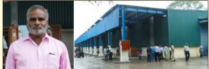
Lean to Roof shed at Furnishing Division was inaugurated by Shri. P.Yuvaraj , Sr.Tech/Shop-88, in the presence of ICF's team of Officers and Staff on 30.10.2017
