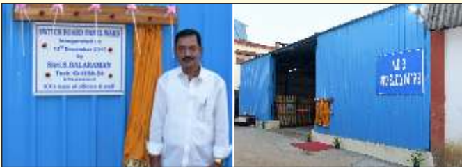
Ward-35, Switch Board Cabinet Shed was inaugurated at Furnishing on 13.12.2017 by Shri. S.Balaraman , Tech-II/54, in the presence of ICF's Team of Officers & Staff.
